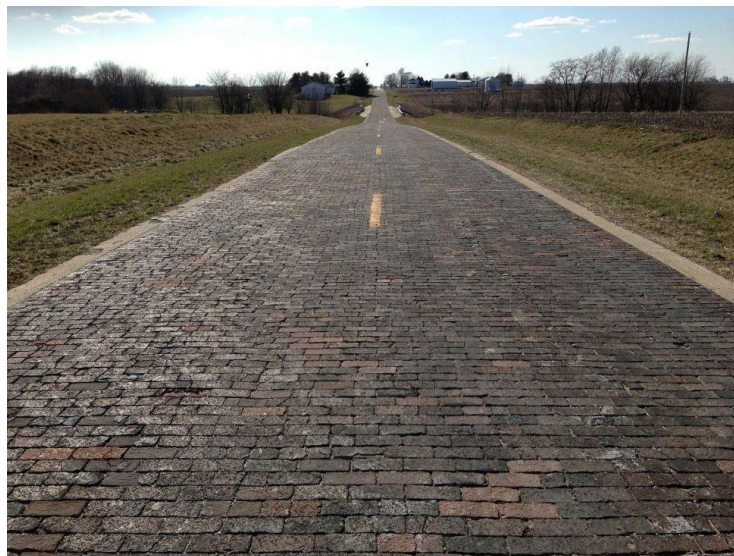
Brick section of Route 66 in Auburn, Illinois. Photo by Jim Grey .
